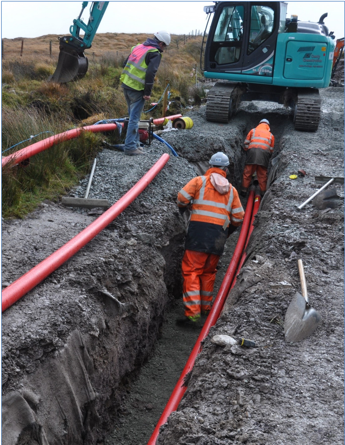
Plate 2: View from NW of linear cable trenching.
